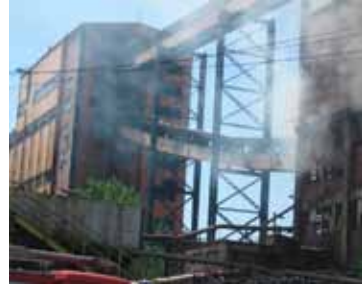
Pict. 6: Fire on conveyor bridges
