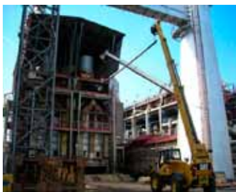
Pict. 11: Oil refinery furnace repair
