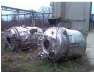
Pict. 9: Vessels after explosion in chemical industry
